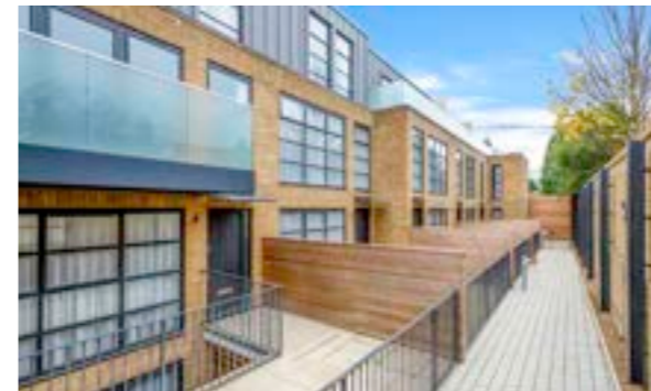
BELLENDEN STUDIOS Six new build flats and two houses in Peckham
